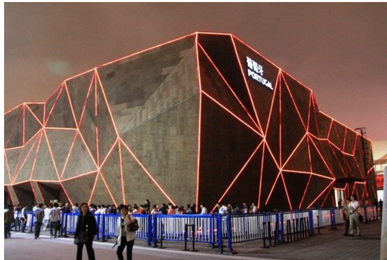
Agglomerate of expanded cork (ICB) - Insulation and external covering (Xangai 2010)
